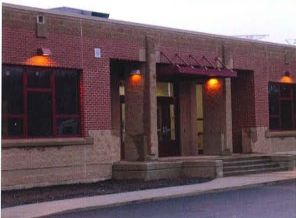
Entrance to administration offices
