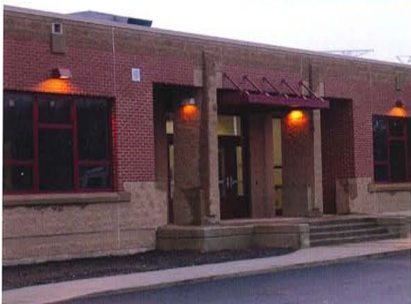
Entrance to administration offices
